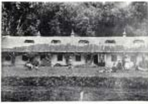
William Bray's "Avonhead" mud wall house
